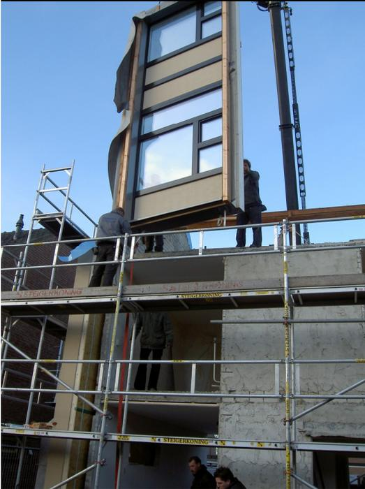
Prefabricated elements are placed after demolition of external layer of the cavity wall.
