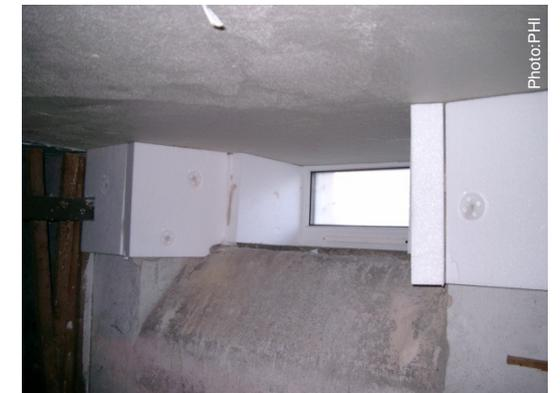
Basement ceiling: The insulation is continued vertically for 30 cm at the interior and exterior walls.  $\Psi_a = 0.30 - 0.46 \text{ W/(mK)}$
