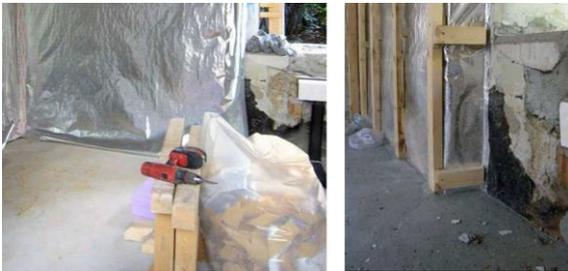
figure 17: Air-tight connection thanks to concrete screed on the floor (c) Manuel Benedikter
