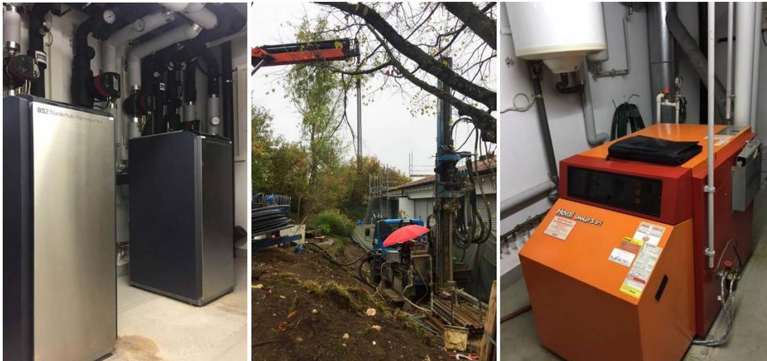
figure 106: From left to right: new geothermal heat pump heating system; execution of the bore holes and oil boiler pre-intervention. © D. Studer
