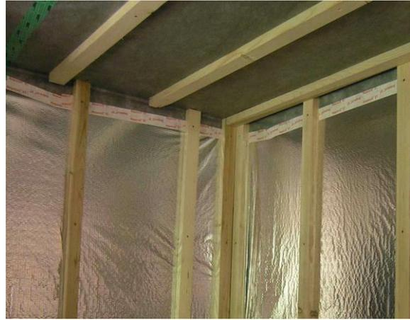
figure 14: Battens for installation layer, which avoids penetrating the vapour barrier with pipes and cables (c) Manuel Benedikter
