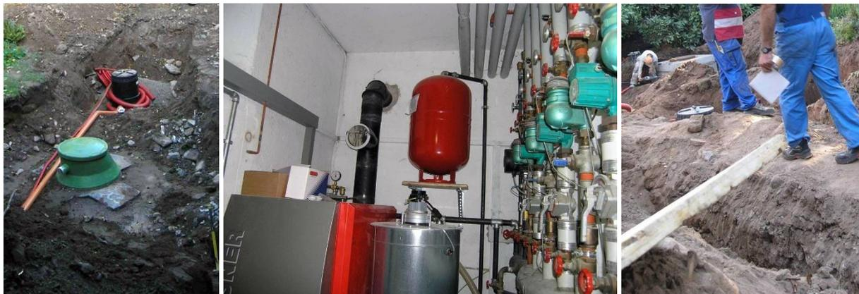
figure 83 Opening of buried pellets tank (left), pellets boiler and distribution (middle) and earth works for pre-heating and cooling ventilation air (right) © Manuel Benedikter Architekt
