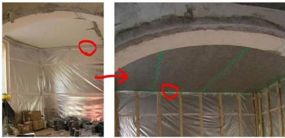
figure 15: © Vapour barrier on the walls and its connection to the vapour retarder in the ceiling (c) Manuel Benedikter
