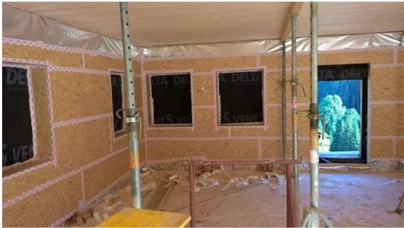
figure 1: airtight layer with glued OSB boards, © DI Hans Peter Gruber
