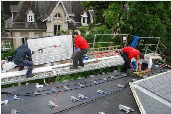
figure 98: Installation hybrid system © M. Hutterli
