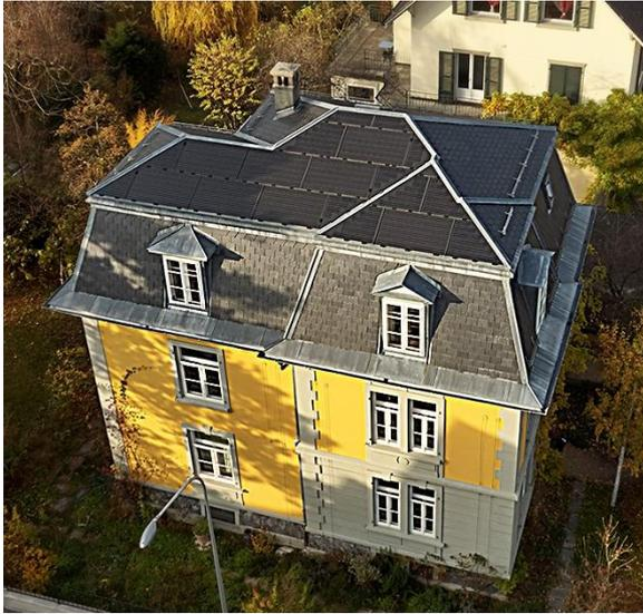
*figure 102: South slope with integrated solar thermal collectors under natural slate roof and BIPV and PVT hybrid modules © C. Martig.*
