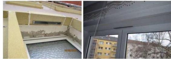
figure 52: © Fraunhofer Institut, Prefabricated box integrating the air inlet before installation of the new window (left) and after (right)
