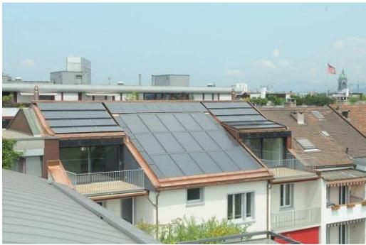
figure 95: Roof with solar thermal and PV ©Nina Mann
