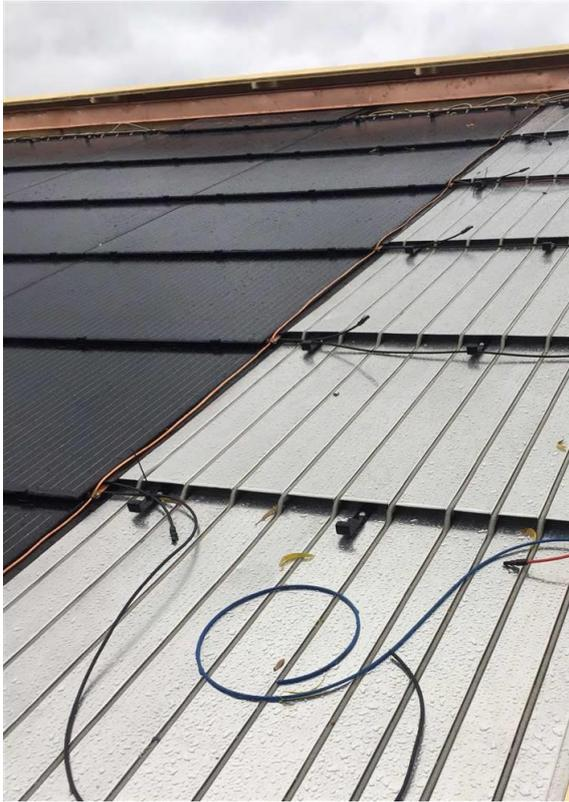
figure 107: PVT panels during works ©Studer
