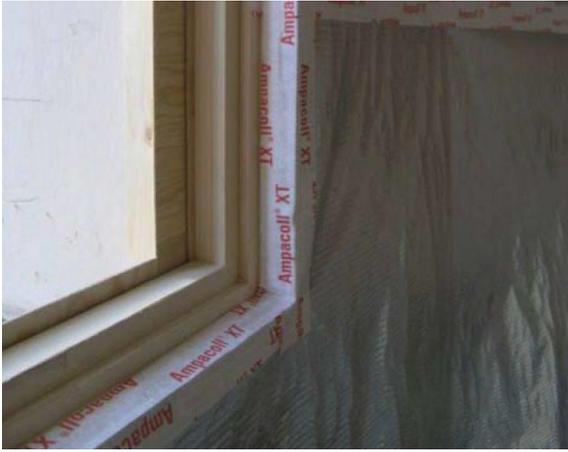
figure 13: Air-tight connection to the window frame (c) Manuel Benedikter
