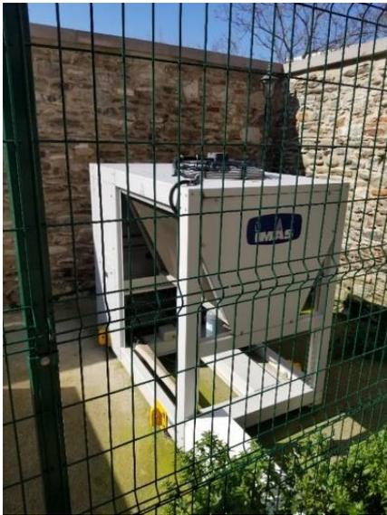
figure 69: Heat pump outdoor unit © IYTE
