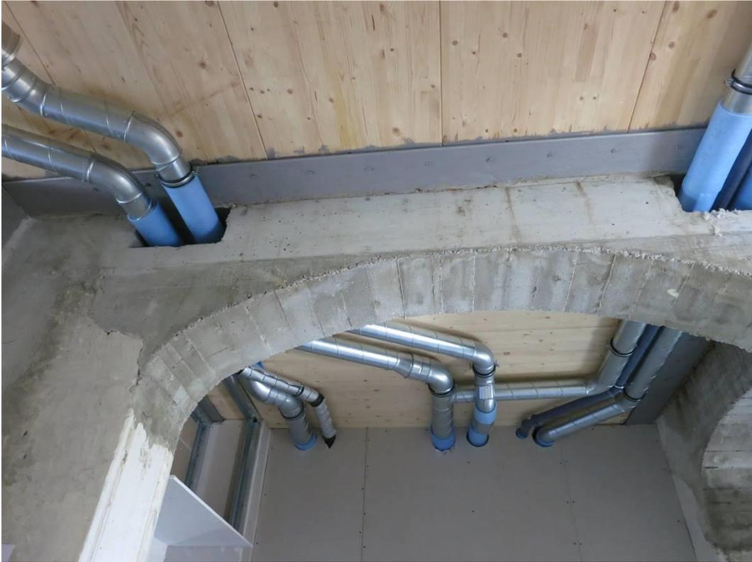
figure 20: Horizontal ventilation distribution / piping, © Valentina Cari
