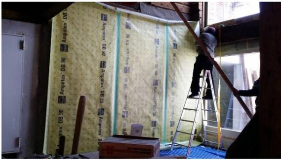
figure 7: vapour barrier and airtight level with Ampatex DB 90 above an internal insulation with sheep wool, © Madritsch und Pfurtscheller Architekten
