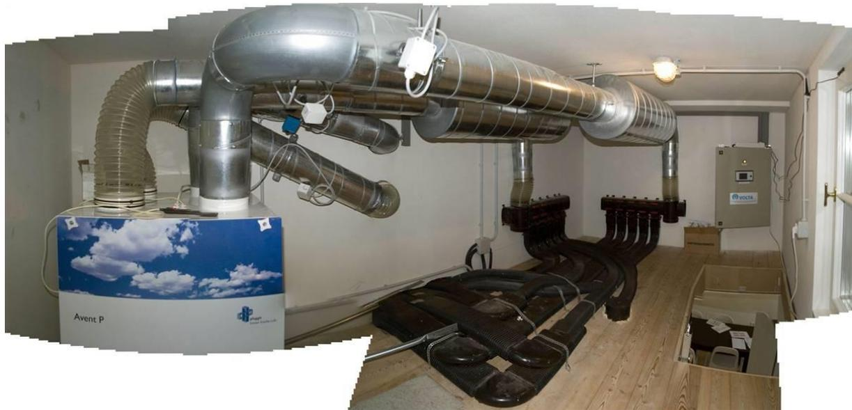
figure 38: Ventilation unit in the crawlspace above the kitchen, © Manuel Benedikter Architekten
