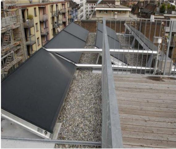
figure 84: Roof view with solar panels ©V+P, Viridén + Partner AG
