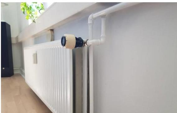
figure 56: Visible piping to/from radiator in apartment (from Denmark), ©Jørgen Rose (SBI)
