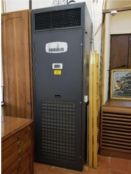
figure 71: Heat pump – indoor unit © IYTE
