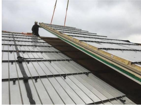
figure 108: PVT panels during works ©Studer
