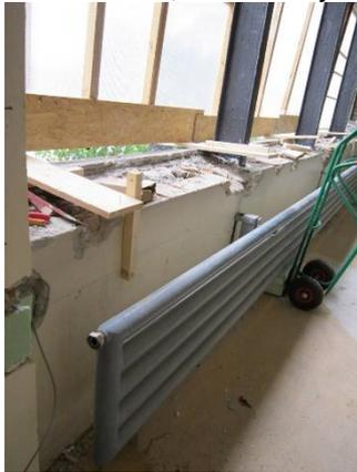
figure 60: Gap between the wall and the radiators for the internal insulation, ©UIBK
