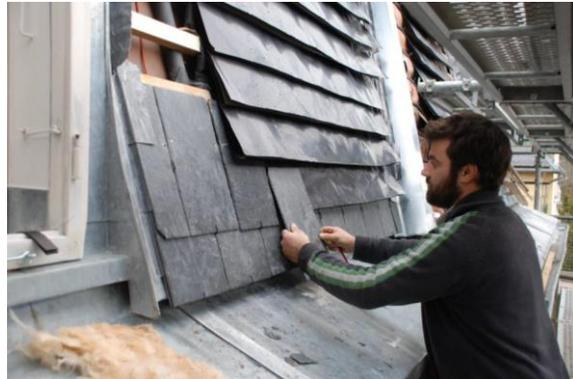
figure 99: Installation slate system © M. Hutterli
