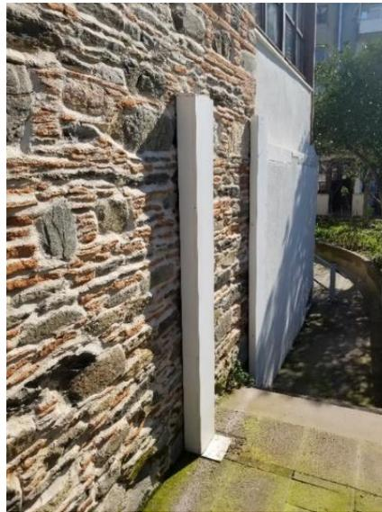
figure 70: Refrigerant line (covered) between indoor and outdoor units of heat pump © IYTE
