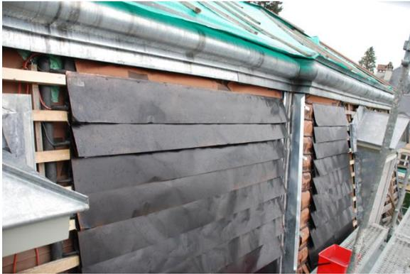
*figure 103: Assembly of during construction works of solar thermal collectors under the natural slate roof. © M. Hutterli*
